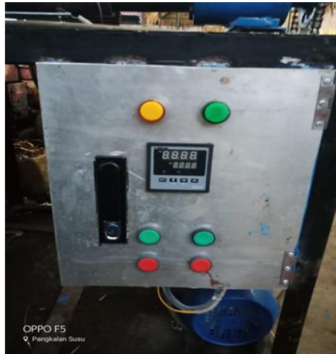
Gambar 3.4 Kontroler suhu (thermostar)
