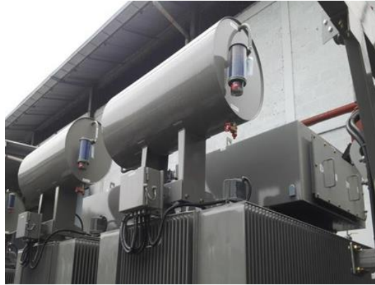
Gambar 2.5 Konservator Oil Preservation And Expansion
