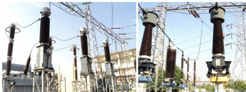
Gambar 2.9 Transformator Arus
