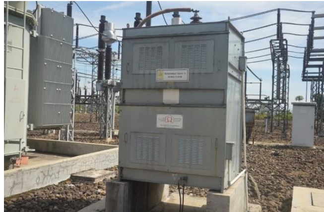
Gambar 2.8 Neutral Grounding Resistor (NGR)
