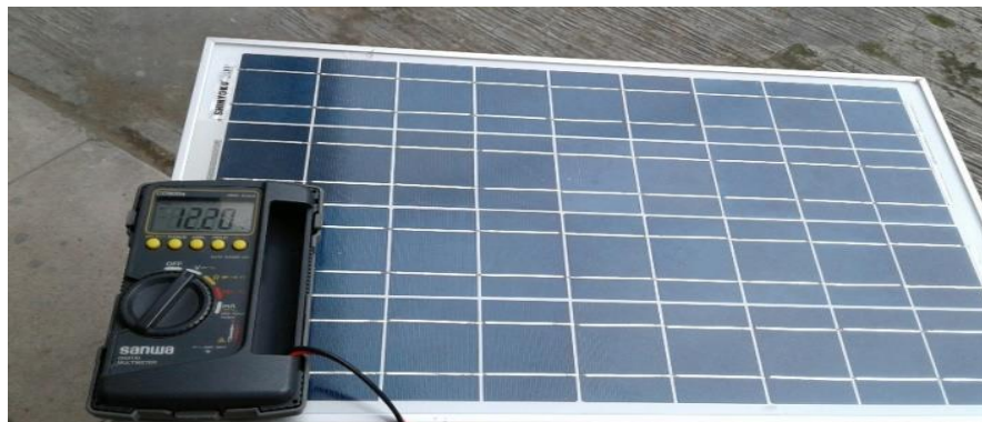
Gambar 4.2 Proses pengukuran tegangan panel surya
