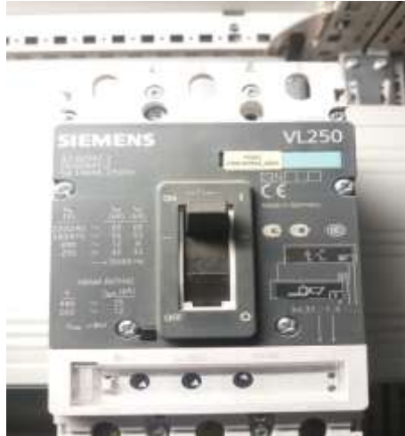
Gambar 2.16 MCCB ( Molded Case Circuit Breakers )
