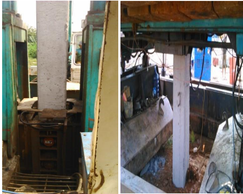
Gambar 2.5: Campling & Piling.
