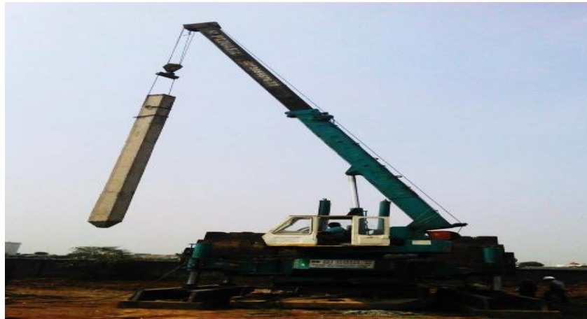
Gambar 2.4: Lifting Pile .
