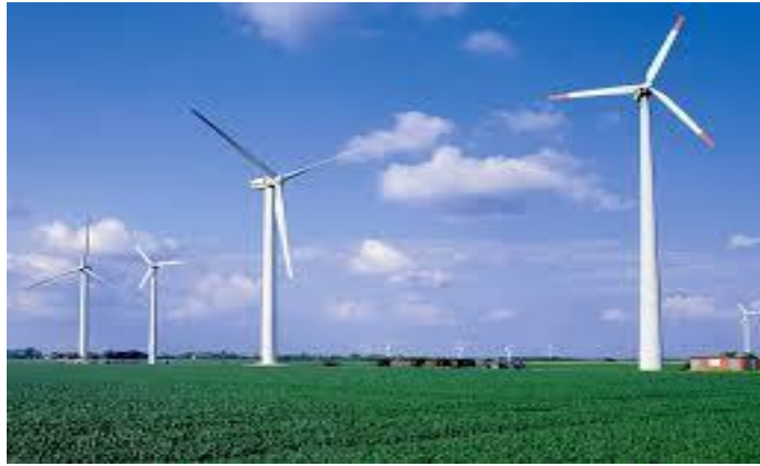
Gambar 2.5 Turbin angin sumbu horizontal (TASH). (Ridomanik 2014)
