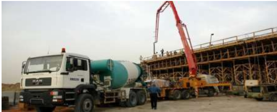
Gambar 4.13: concrete pump (PT. Wijaya Karya (persero) Tbk ).
