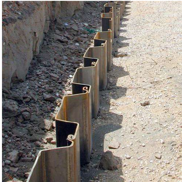
Gambar 2.11 Dinding Steel Sheet Pile
