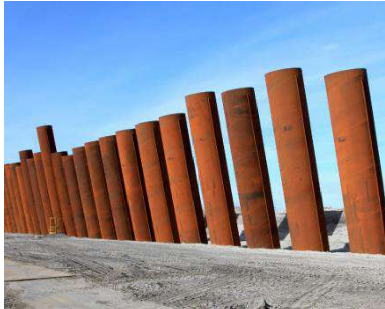
Gambar 2.12 Tubular Pile
