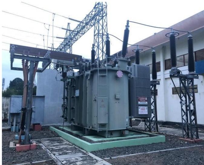
Gambar 2.1 Transformator Daya (GI PLN Glugur)
