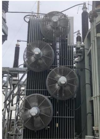
Gambar 2.11 Pendingin Transformator Daya (GI PLN Glugur)
