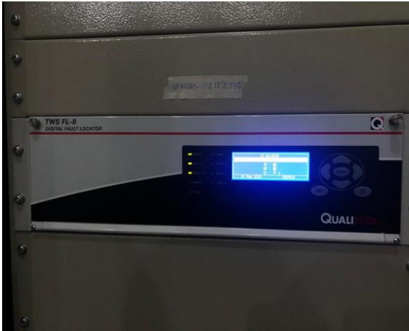
Gambar 3. Fault Locator
