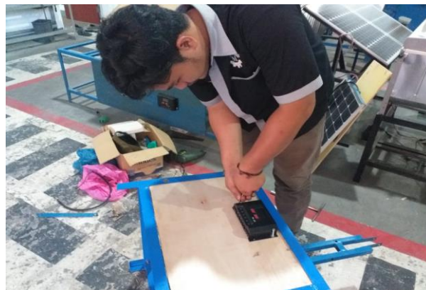
Gambar 3.26 Memasang Charger Controller
