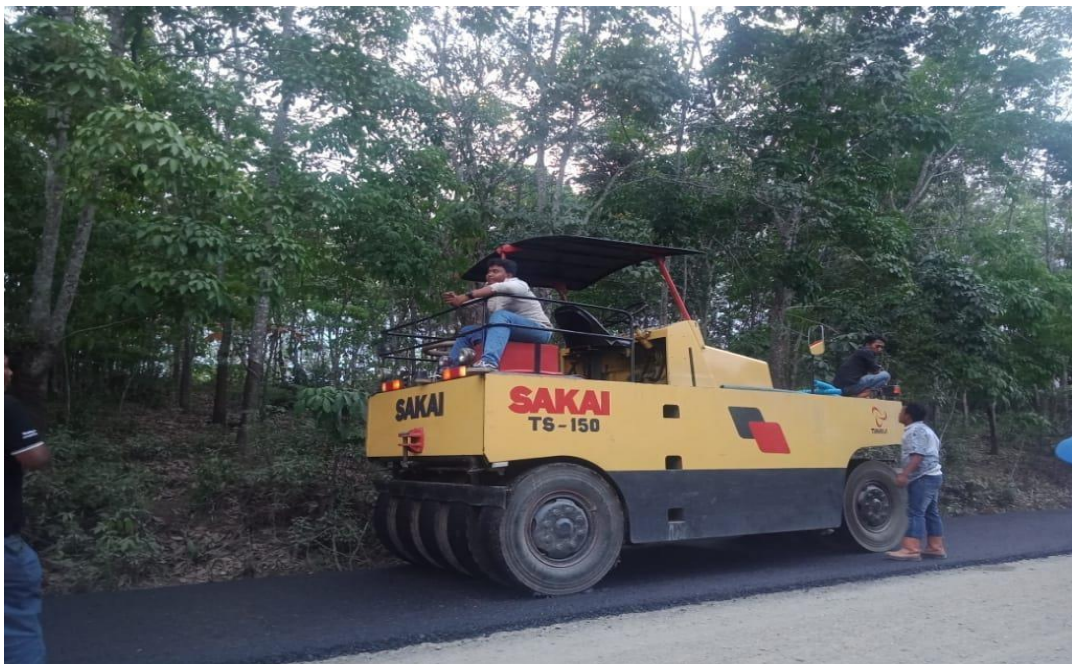
Gambar 6: Pneumatic Tyre Roller saat melakukan pengilasan aspal AC BC
