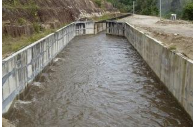
Gambar 2.4 Bak pengendap ( Settling Basin )
