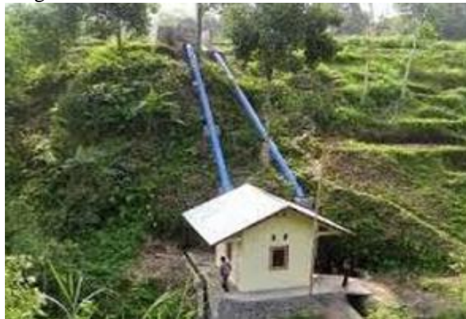
Gambar 2.7 Pipa pesat ( Penstock )
