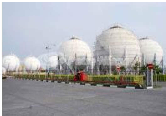
Gambar 2.6 Spherical tank (avturblog.blogspot.com)
