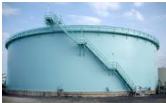
Gambar 2.4 Fixed roof tank
