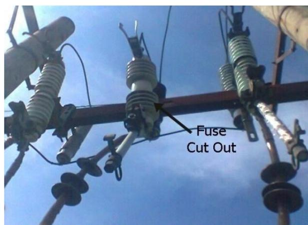
Gambar 2.13. Pemutus Beban 20 KV Tipe “*Fuse Cut Out*”
