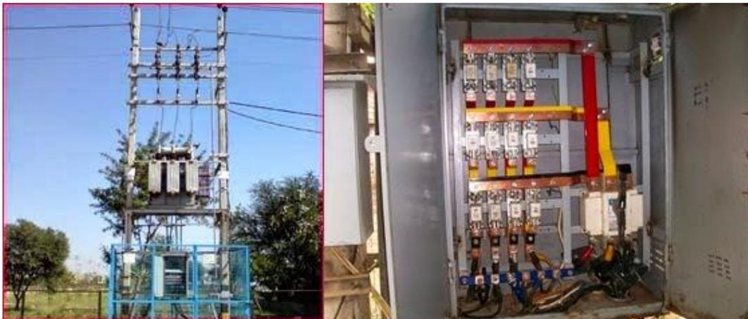
**Transformator distribusi 315 KVA + Low Voltage Cabinet ( LVC )/**
