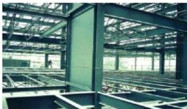
Gambar 2.9: *Steel plate shear walls* (Seilie dan Hooper, 2005).
