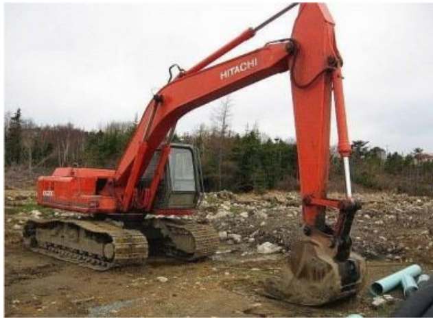
Gambar 2.1 Excavator Hitachi Ex200
