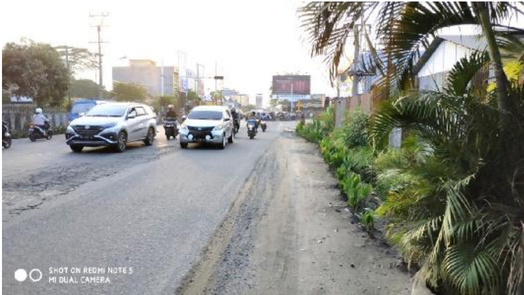
Gambar L3: Jalan Medan-Binjai Km 12
