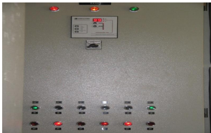
GambarPanel Box Kapasitor Bank
