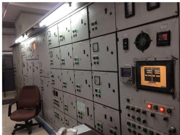
Panel Kontrol Boiler Mckenzie Berkapasitas 40 Ton
