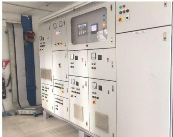
Panel Kontrol Boiler Combi Berkapasitas 30 Ton
