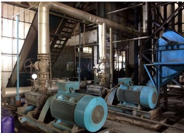
Motor Feed Pump Boiler Mckenzie Berkapasitas 40 Ton
