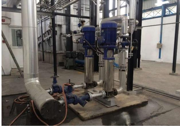
Motor Feed Pump Boiler Combi Berkapasitas 30 Ton
