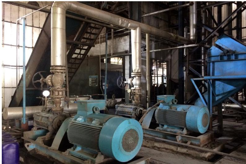
Gambar 3.3 Motor Feed Pump
