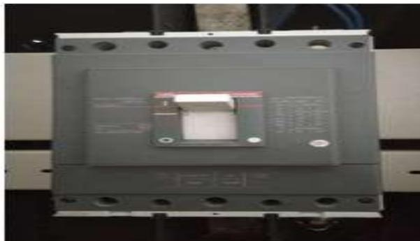
Gambar2. 8 MCCB (Molded Case Circuit Breaker)
