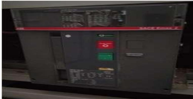
Gambar2. 9 ACB (Air Circuit Breaker)
