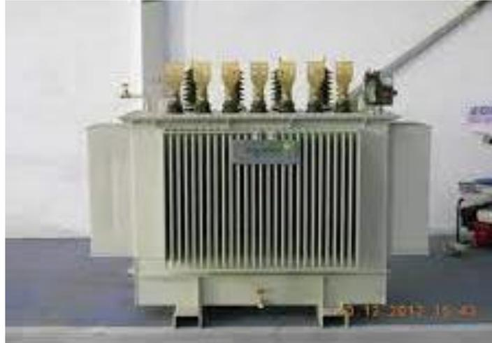
Gambar2. 11 Trafo Distribusi (Distribution Transformer)
