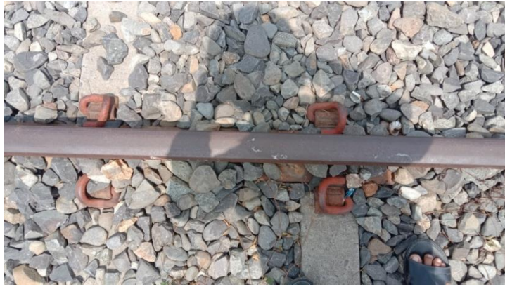
Gambar 9 . Bantalan,Rel,Ballast,Penambat Pandrol (EG)
