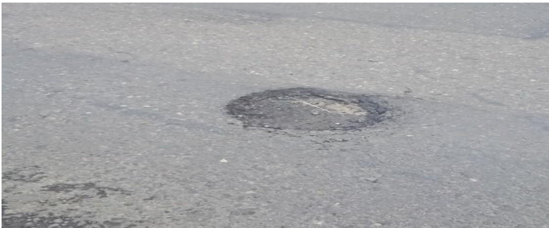
Gambar 2. 15 : Lubang (dpu.kulonprogokab n.d.)
