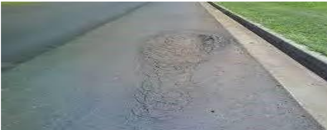
Gambar 2. 12 : Sungkur (Shoving)(dpu.kulonprogokab n.d.)
