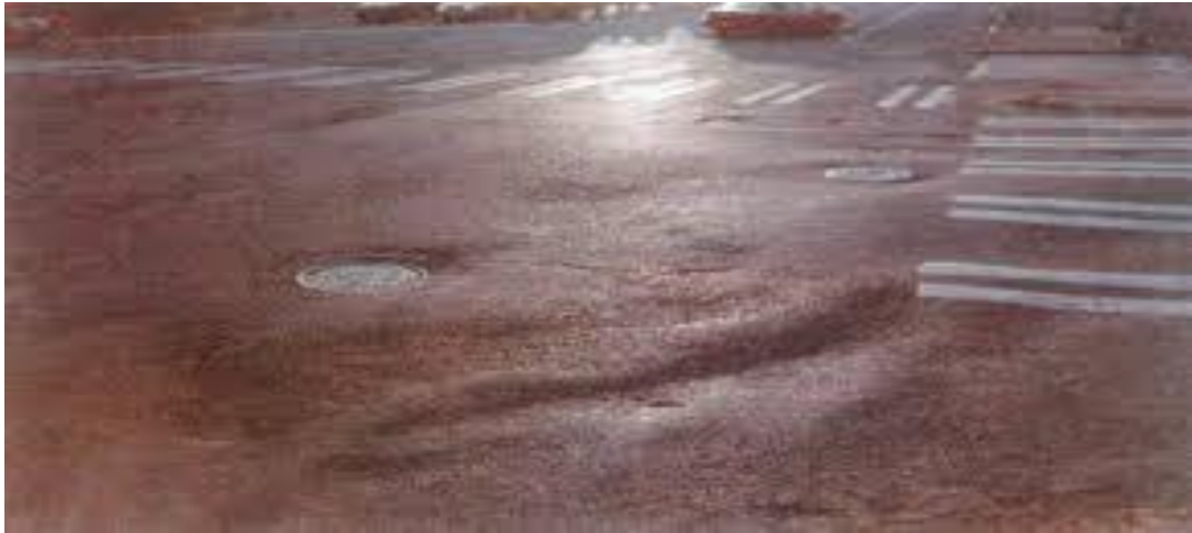
Gambar 2. 11 : Keriting (dpu.kulonprogokab n.d.)
