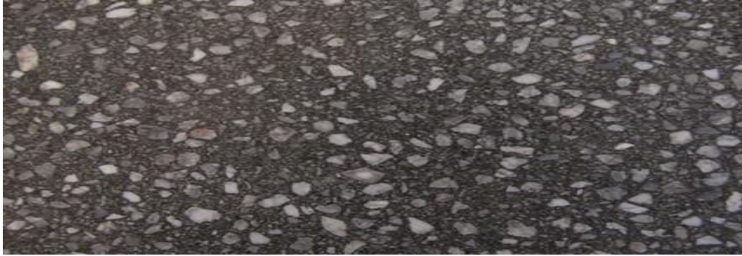
Gambar 2. 18 : Pengausan (Polished Aggregate) (dpu.kulonprogokab n.d.)
