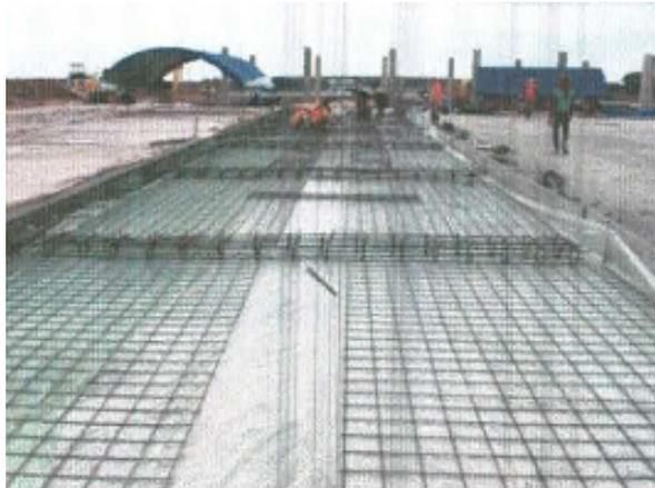
Gambar L2: Pemasangan wiremesh.
