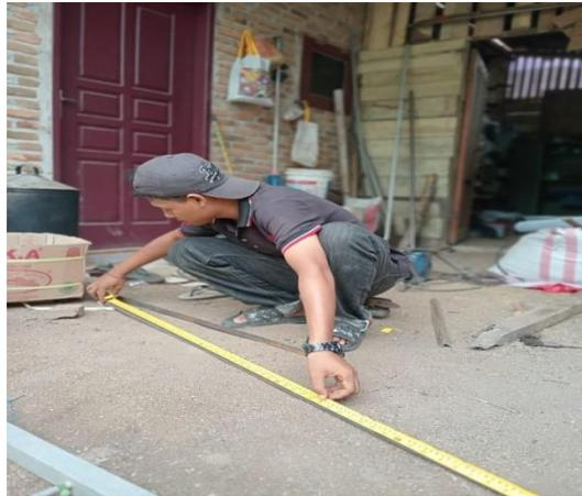
Gambar 4. 1 Mengukur besi hollow
