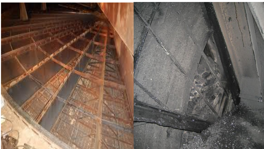
Gambar 4.8 Elemen heat Air Preheater
