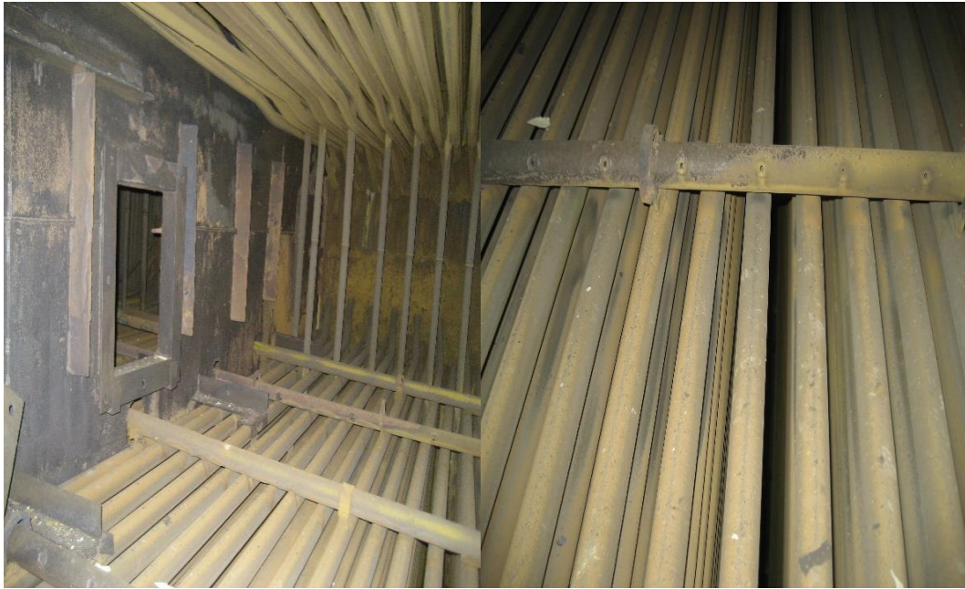
Gambar 4.5 Tube-tube Secondary Superheater
