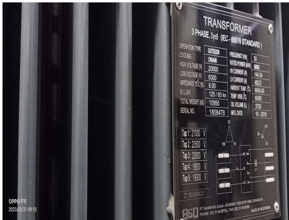
Gambar 3. 1 Transformator 5000 kVA
