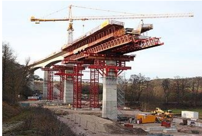
Gambar 2. 2 : Movable Scaffolding System.
