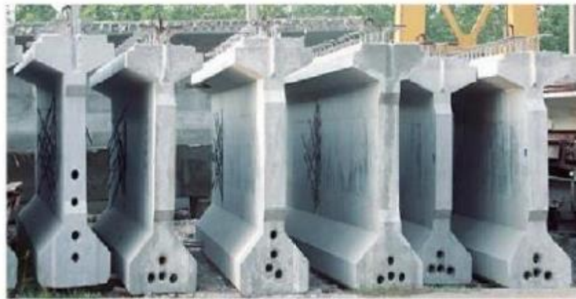
Gambar 2.5: Gelagar Beton Prategang
