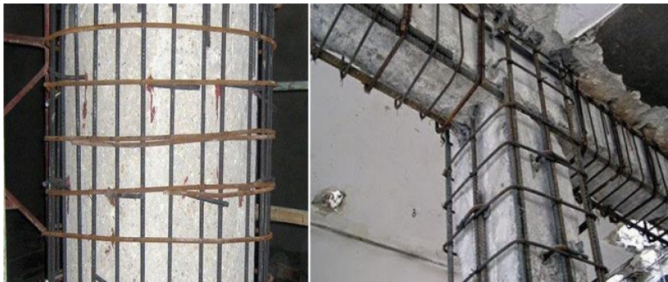
Gambar 2.6: Jacketing Concrete.
