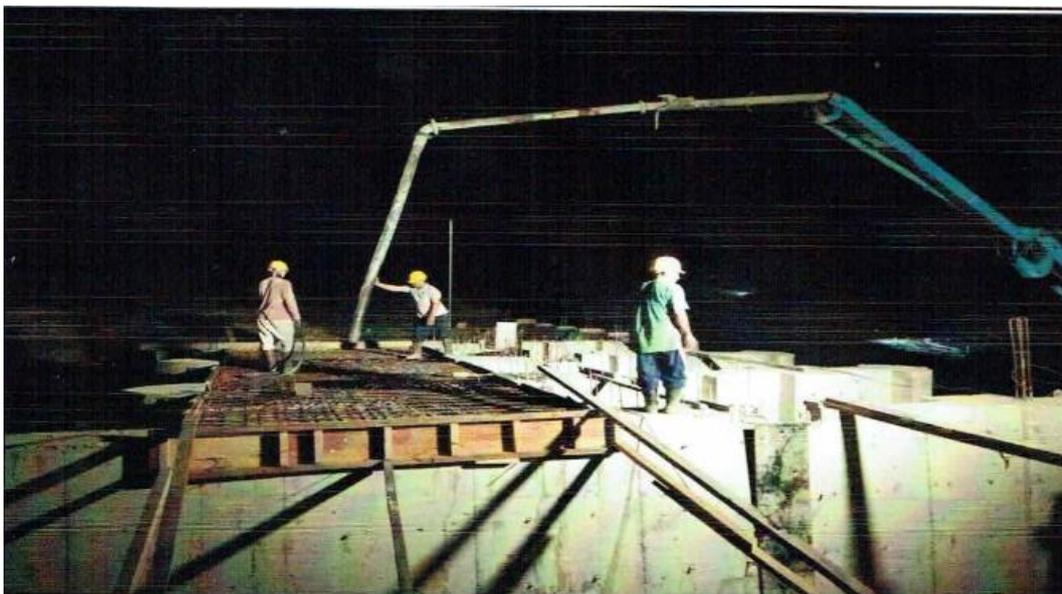
Gambar 3.3: Pengecoran beton mutu K300.
