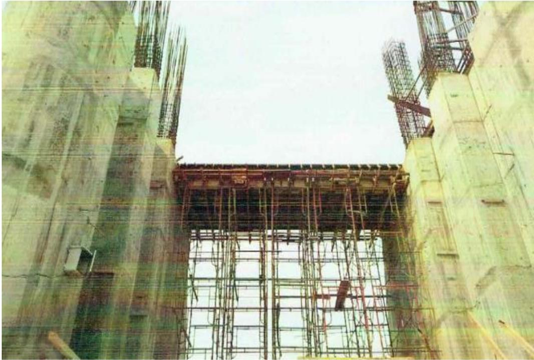
Gambar L1: Pemasangan Bekisting.
