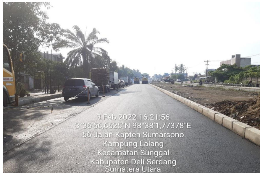
Gambar L.6: Lapisan perkerasan AC-WC
