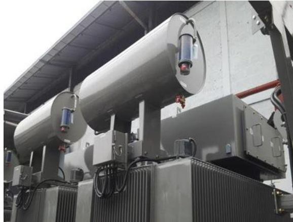
Gambar 2.7 Konservator Oil Preservation and Expansion
