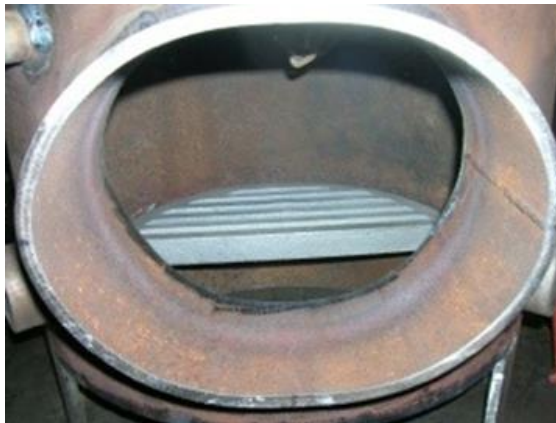
Gambar 2.6 Ruang Bakar ( furnace ) (Sumber: Apit Fathurohman, S. Pd., 2015)
