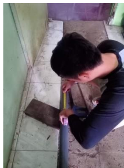
Gambar 4.24 Mengukur Pipa PVC
