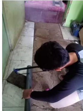
Gambar 4.25 Memotong Pipa PVC
