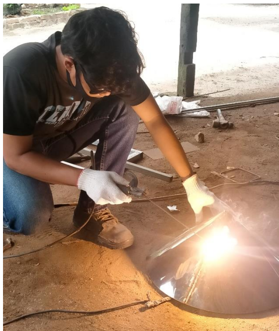
Gambar 4.10 Pengelasan plat stainless
