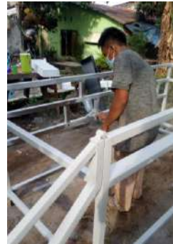
Gambar 4.80. Pengecatan epoxy
