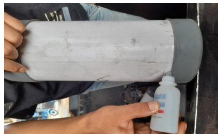
Gambar 4.30 pengeliman pipa
