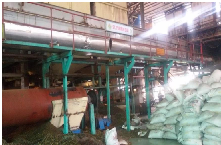
Gambar 2.23 Stasiun Pengolahan Biji ( Nut Plant Station )
