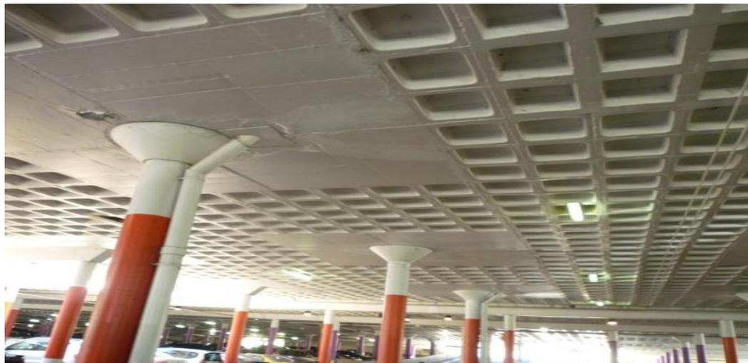
Gambar 2.10: Konstruksi *Waffle Slab* (Paul, 2014).
