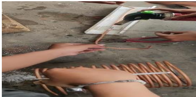
Gambar 4.7 Pengelasan Helical Coil
