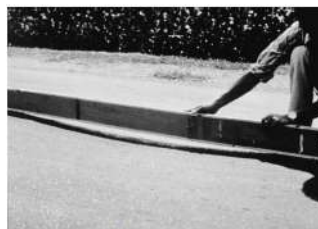
FIG. X1.17 Medium-Severity Depression
