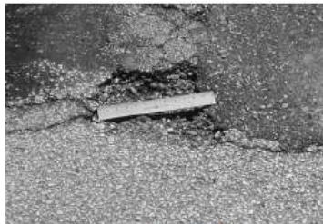
FIG. X1.35 Low-Severity Pothole
