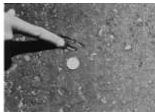
FIG. X1.5 Medium-Severity Bleeding
