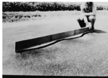
FIG. X1.15 High-Severity Corrugation
