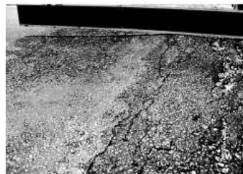
FIG. X1.12 High-Severity Bumps and Sags
