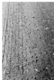
FIG. X1.6 High-Severity Bleeding
