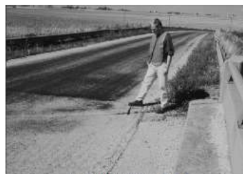
FIG. X1.44 Low-Severity Shoving
