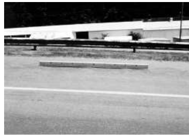
FIG. X1.14 Medium-Severity Corrugation
