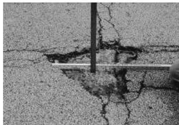
FIG. X1.36 Medium-Severity Pothole
