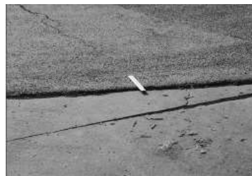
FIG. X1.45 Medium-Severity Shoving
