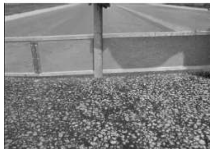
FIG. X1.42 Medium-Severity Rutting
