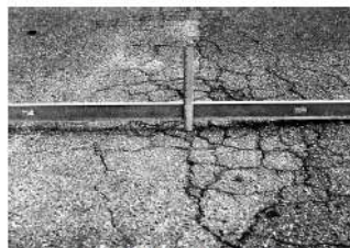
FIG. X1.18 High-Severity Depression
