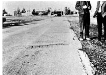
FIG. X1.11 Medium-Severity Bumps and Sags
