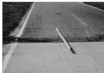
FIG. X1.46 High-Severity Shoving
