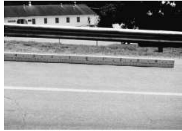
FIG. X1.13 Low-Severity Corrugation
