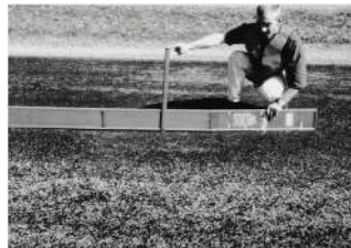
FIG. X1.16 Low-Severity Depression
