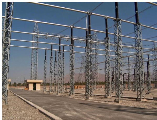
Gambar 2. 13 Rel Busbar
