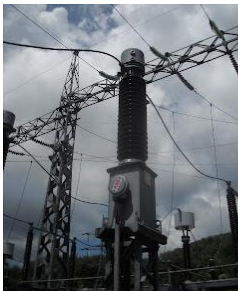
Gambar 2. 10 Transformator arus
