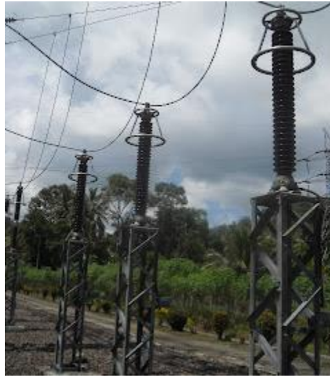
Gambar 2. 9 Lightning Arrester (LA)
