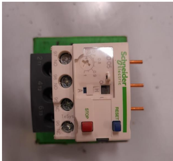
Gambar 2.21. Thermal Overload Relay
