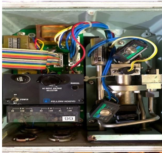
Gambar 2.5 Sensor Kadar Minyak (Oil Content Monitor/OCM)
