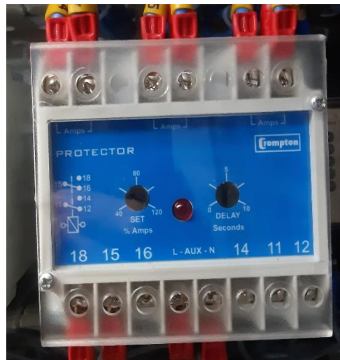
Gambar 2.6. Fisik Rele Arus Lebih ( Over Current Rele )
