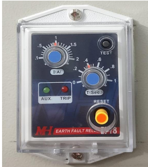
Gambar 2.10. Fisik Rele Gangguan Tanah ( Earth Fault Relay )
