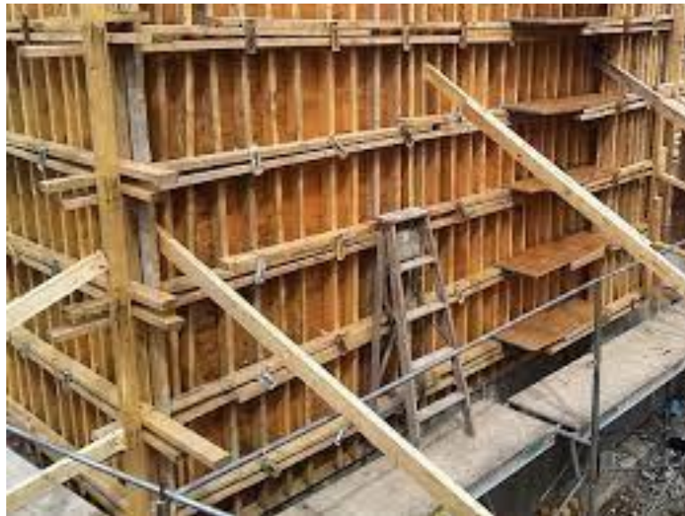
Gambar 2.1: Bekisting Konvensional
