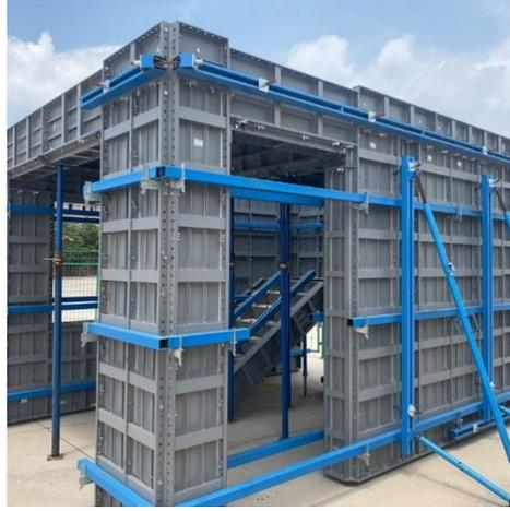
Gambar 2.13: Bekisting Aluminium.
