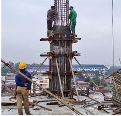
Gambar 2.11: Bekisting Semi Sistem.
