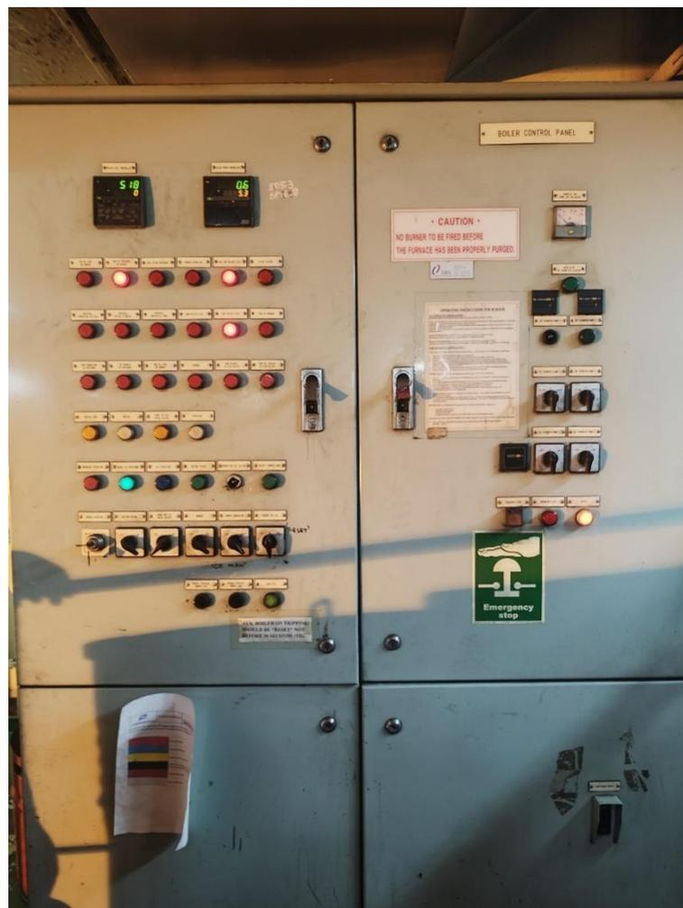
Gambar 2. 15 Panel *Control* Boiler
