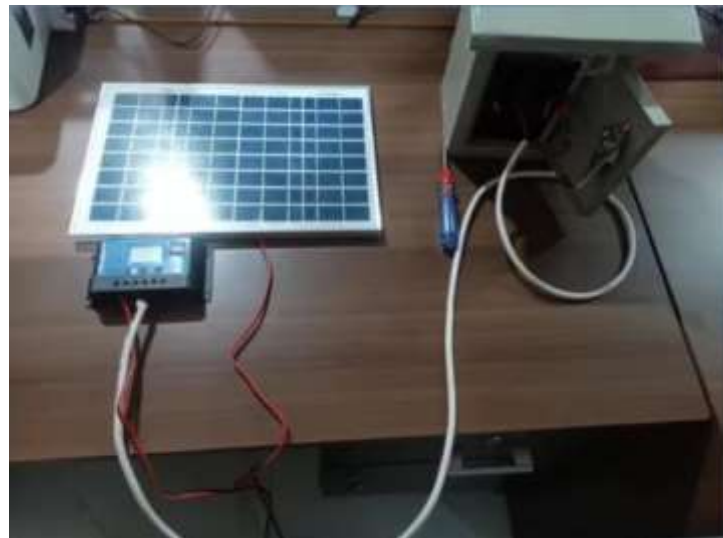
Gambar 4.5 Proses instalasi solarpanel Gambar
